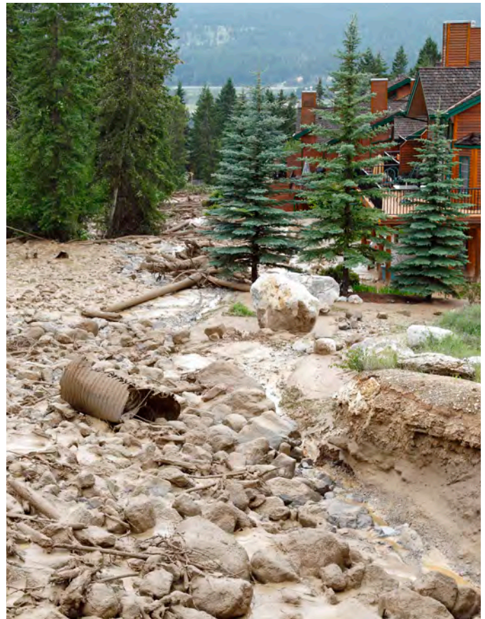
Mud slide with rock, boulders, and debris
